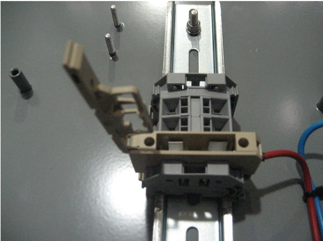
Illustration shows the fuse holder open with no fuse fitted
